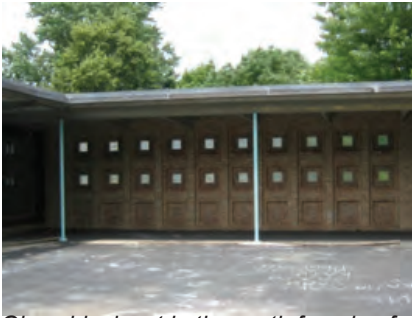
Glass block set in the north façade of play terrace, northwest wing (BHC)
