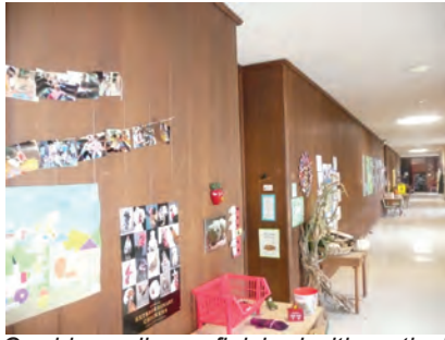
Corridor walls are finished with vertical pine planks with v-grooves (BHC)
